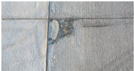
**SPALLING.** Spalling, in PCC pavement, is the breakdown of the slab edges near the slab joint. Spalling is identified as occurring in the corner or along the joint of a PCC slab. Spalling is typically caused by the introduction of incompressible material in the joint, weaker pavement at the joint caused by overworking of the pavement during construction, traffic loading or a combination of these.
