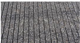
**WEATHERING.** As pavements age and are exposed to oxidation and other environmental stresses, they may experience a loss in the material making up the pavement matrix. Weathering is the loss of asphalt binder and fine aggregate in the surface of the pavement. The loss of fine matrix material in the surface may eventually lead to the exposure and dislodging of coarse aggregate, leading to raveling and FOD.
