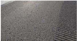
**RAVELING.** As pavements age and are exposed to oxidation and other environmental stresses, they may experience a loss in the material making up the pavement matrix. Raveling is the dislodging and loss of coarse aggregate in the surface of a pavement. The pavement may be showing signs of aging and hardening and may result in the production of FOD.
