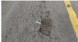
**ALLIGATOR CRACKING.** Alligator (fatigue) cracking is a load-related distress caused by excessive tensile strains at the bottom of the AC layer or stabilized asphalt base layer from repeated aircraft loadings. Alligator cracking typically shows up on the surface as a series of parallel cracks, which eventually interconnect to form a pattern resembling the skin of an alligator.
