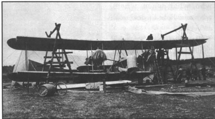
Vickers Vimy being assembled at St. John's, Newfoundland, 1919.
