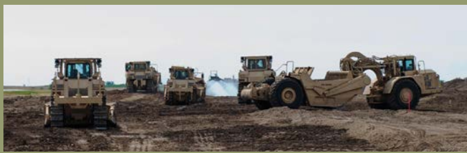
Heavy equipment operators from Detachment 1, 815th Engineer Company (Horizontal), based in Wishek, use bulldozers and a scraper June 12, 2017 to complete groundwork on an apron expansion at the Wishek Municipal Airport. The unit used its 2-week “annual training” period to provide assistance to the Wishek community through a National Guard State Civil-Military Construction Project. (U.S. Army National Guard photo by Spc. Kristin Berg, 116th Public Affairs Detachment/Released)
