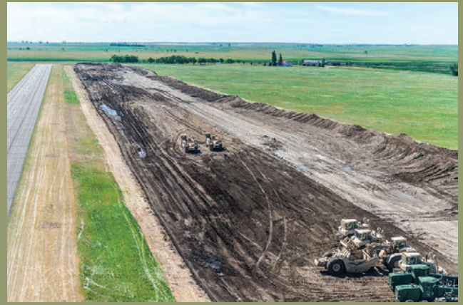
Soldiers from Detachment 1, 815th Engineer Company (Horizontal), based in Wishek, use heavy equipment June 15, 2017 to construct a new taxiway at the Wishek Municipal Airport. The unit used its 2-week “annual training” period to provide assistance to the Wishek community through a National Guard State Civil-Military Construction Project. (U.S. Army National Guard photo by Mr. Jonathan Haugen, N.D. National Guard Visual Information Office/Released)
