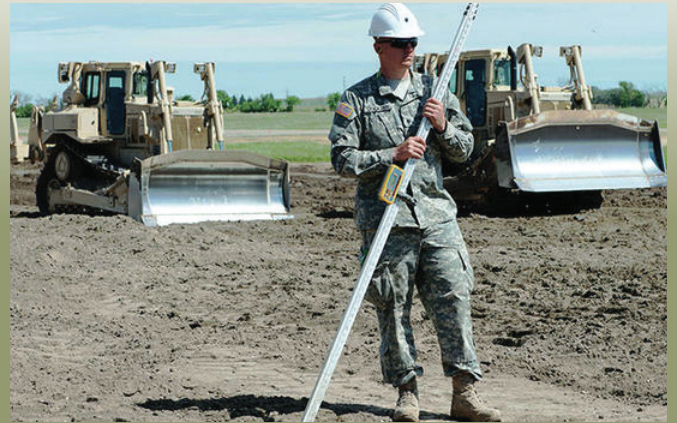
Spc. Drew Docktor, of Valley City, North Dakota, a heavy equipment operator with the 815th Engineer Company (Horizontal), uses a grid stick to make sure dirt is level June 12, 2017, as other soldiers from his unit build a new taxiway at the Wishek Municipal Airport. (U.S. Army National Guard photo by Spc. Thea Jorgensen, 116th Public Affairs Detachment/Released)
